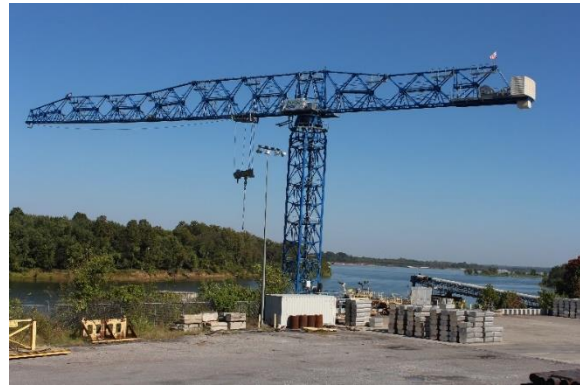
Figure 11: Largest flat top 53-ton crane in North America
